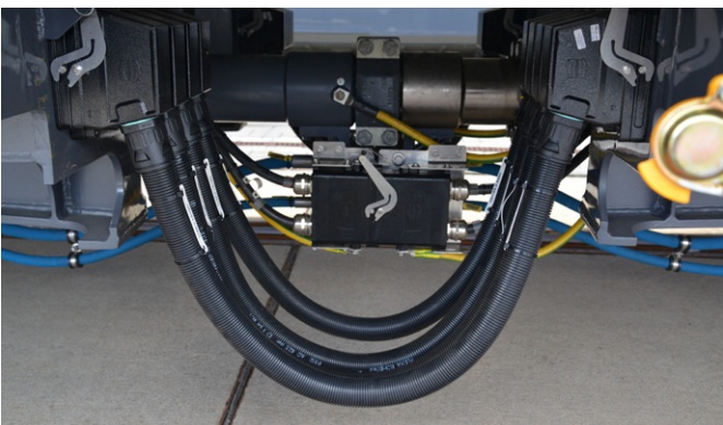
Jumper cable installation
