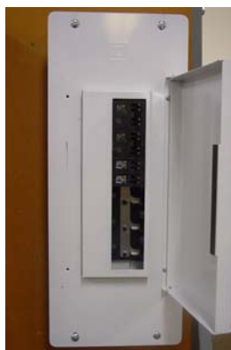
Step #3 Install New HFLCI
